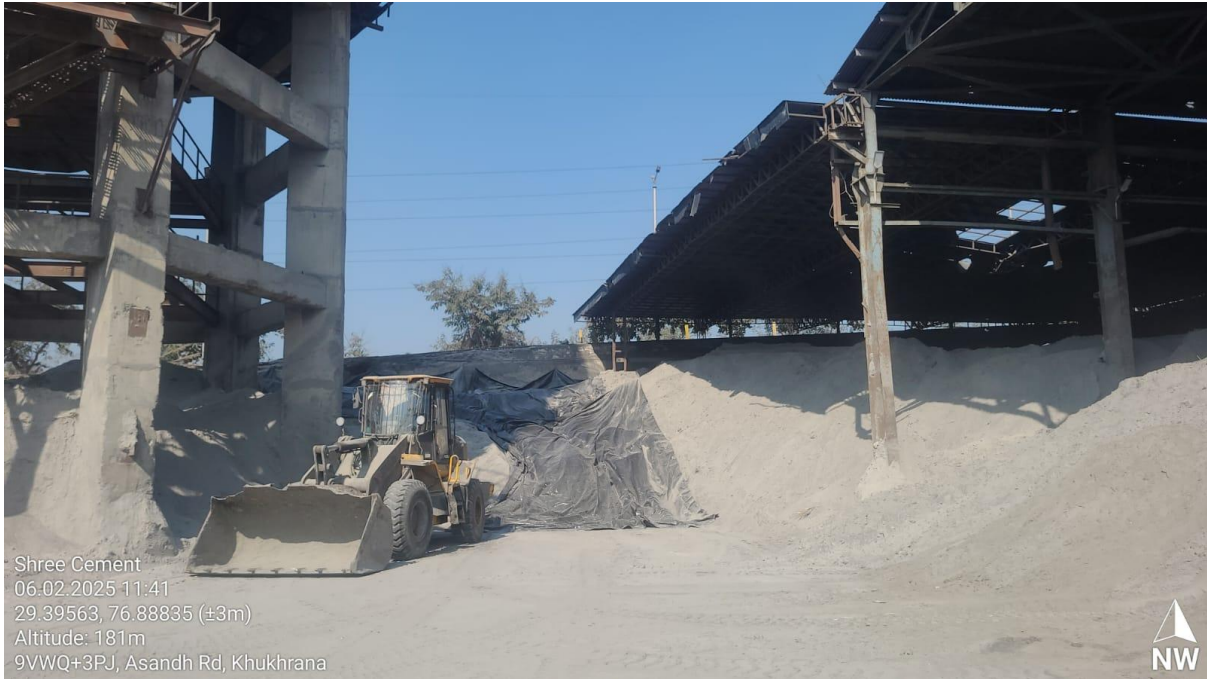
Photograph 5: Pond Ash Storage Area
