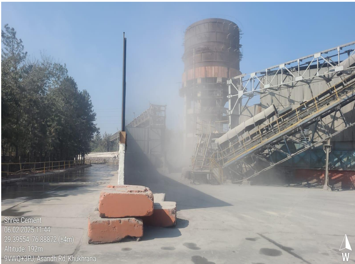
Photograph 6: Dust in Pond Ash Handling Area
