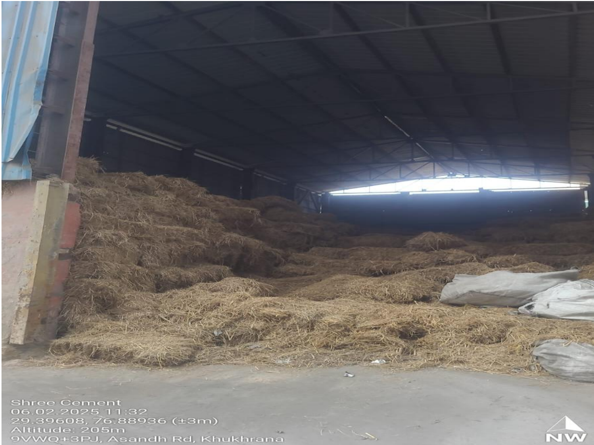
Photograph 7: Biomass fuel stored in covered shed
