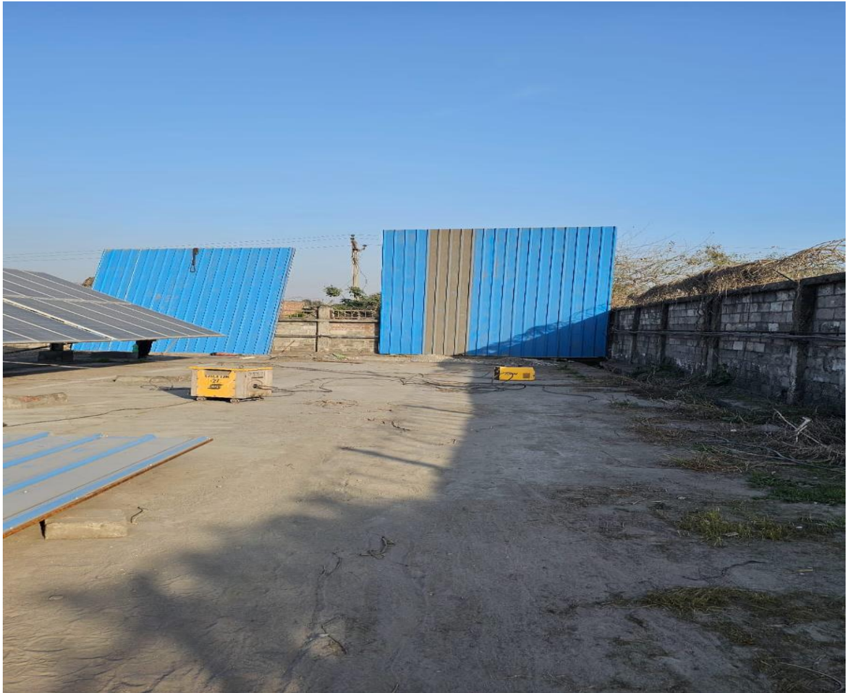
Photograph 9: Wind breaking wall towards village under construction
